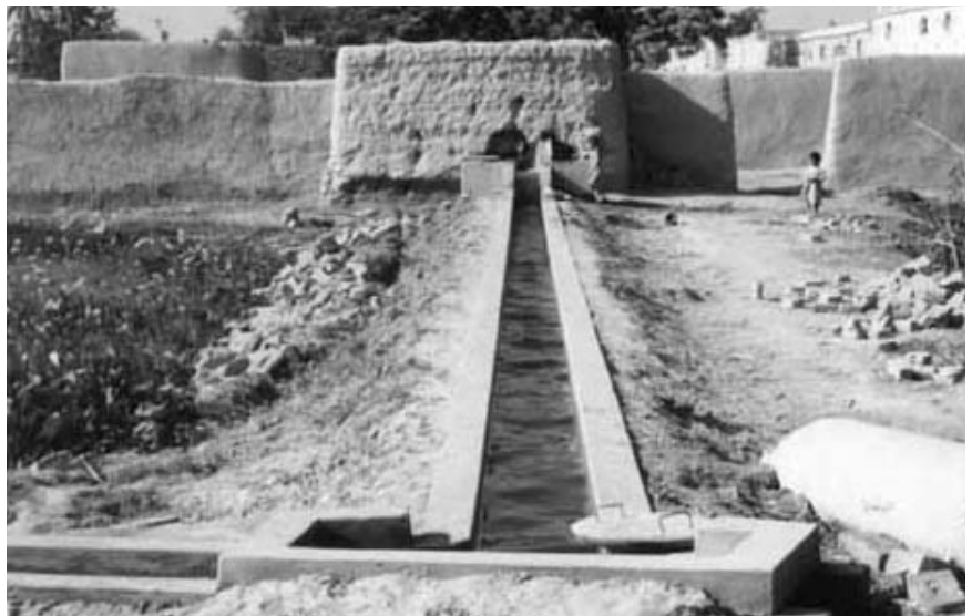
Districts with poor infrastructure deserve greater resources.
